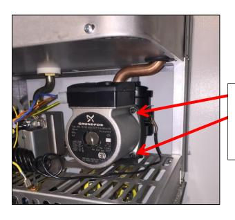
Remove 4 Allen bolts to remove motor from housing
