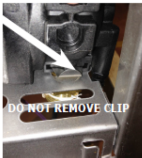
RIGHT SIDE CLIP - INSIDE BOILER JACKET
