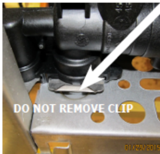
LEFT SIDE CLIP - INSIDE BOILER JACKET
