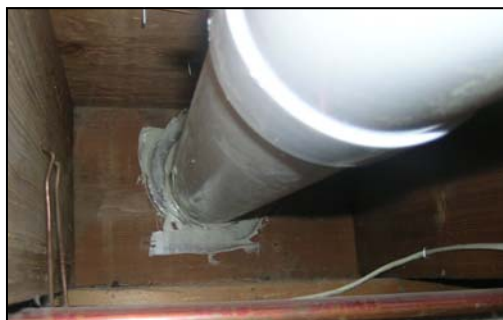
PHOTO 4: Wall penetration
